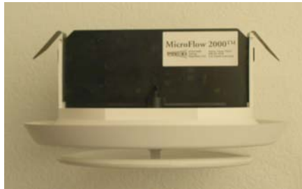
Figure 6 - Manual Air Valve Assembly
