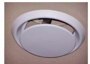
Figure 8 - Installed Register
